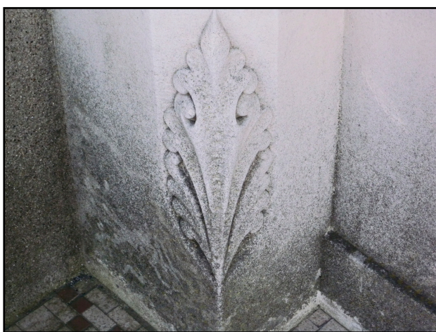
Acanthus leaf detail carved into the base of the pillar flanking the porch door at Roebuck Castle.
